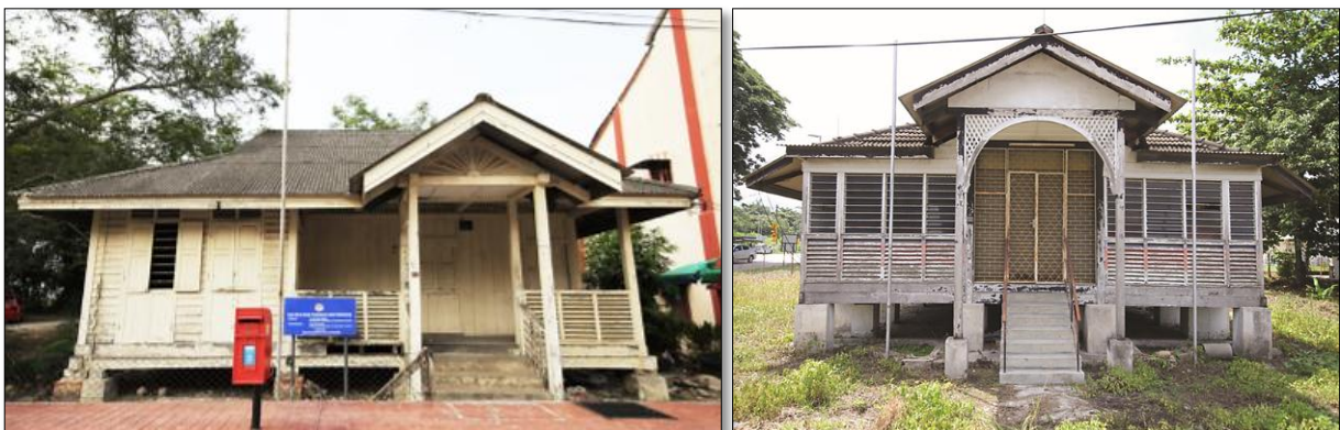
Existing conditions of the abandoned Bagan Datuk Post Office (left) and Tanjung Rambutan Post Office (right).
