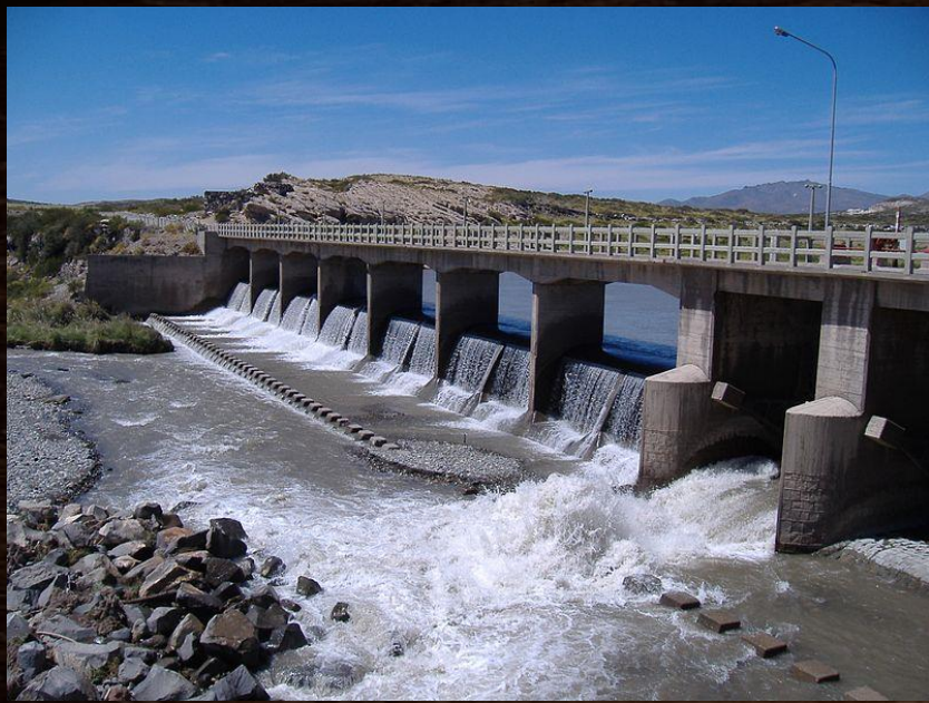
Blas Brisoli Dam, Argentina
